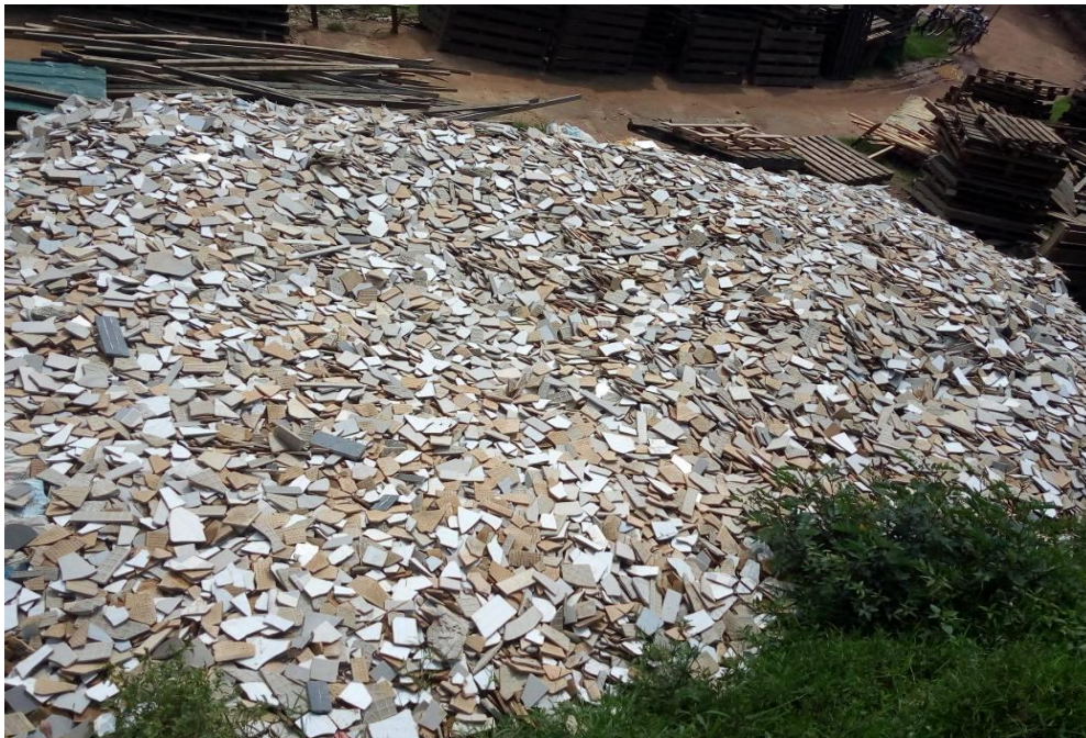
figure.4. 9. Shows the broken ceramic tiles disposed on site which is harmful to the environment
