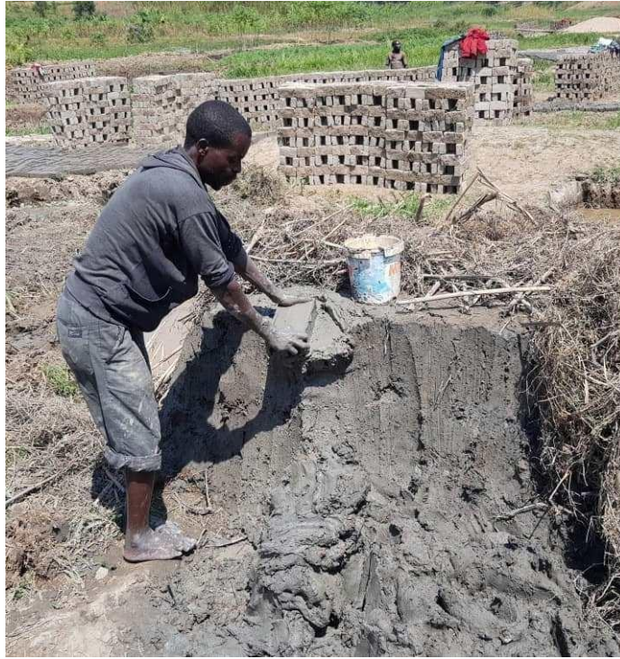
Figure 2.4: Hand moulding of clay bricks
