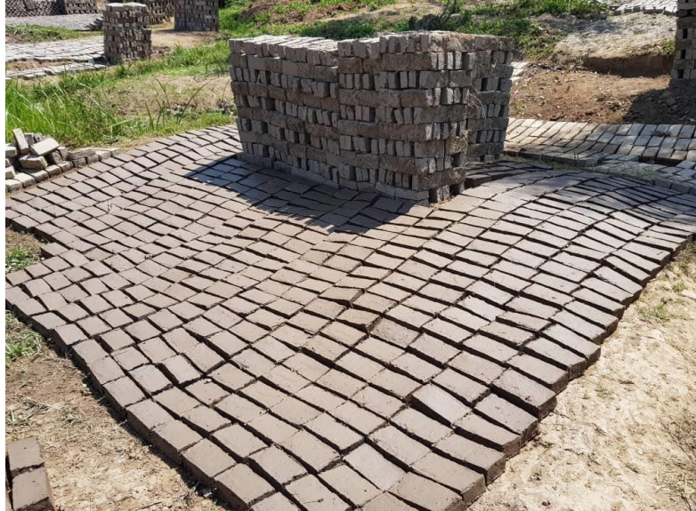
Figure 2.5: drying of clay bricks on the sun
