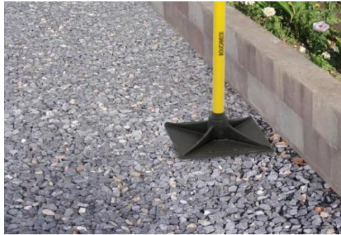
Figure 6.2. Hand compaction
