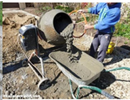
Figure 5.2. Machine mixing
