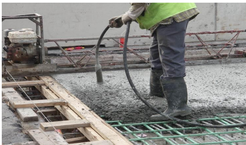
Figure 7.2. Machine compaction
