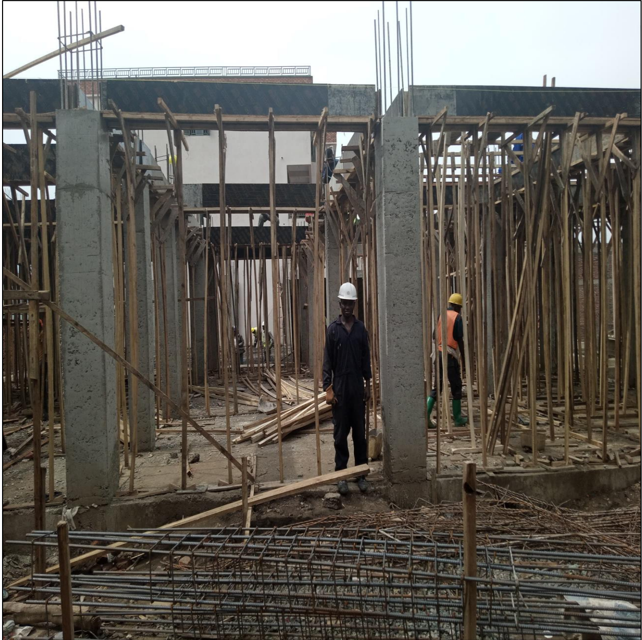
Picture 1: construction of G+2 commercial building at Kimironko sector
